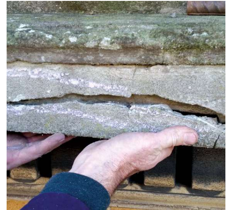
Removal of loose stone during a Safety Audit
