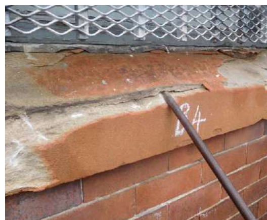
Top image: Block B following facade repairs
