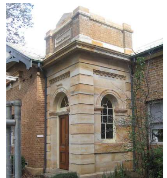
Top image: The sandstone entry was originally sourced from a local quarry Lower image: Detail of the stone entry
