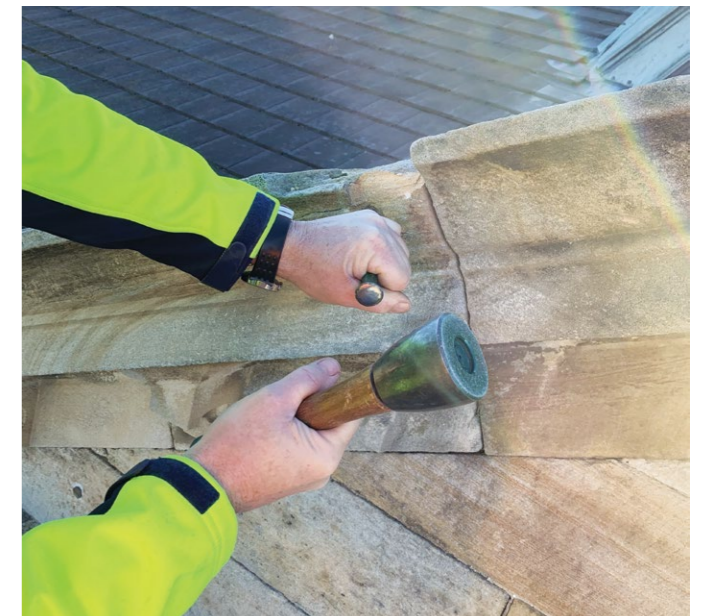
Top right image: Loose, cracked stonework being removed during an inspection.
