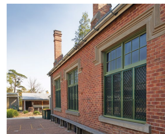
Top image: Greta Public School Lower image: Completed window repairs
