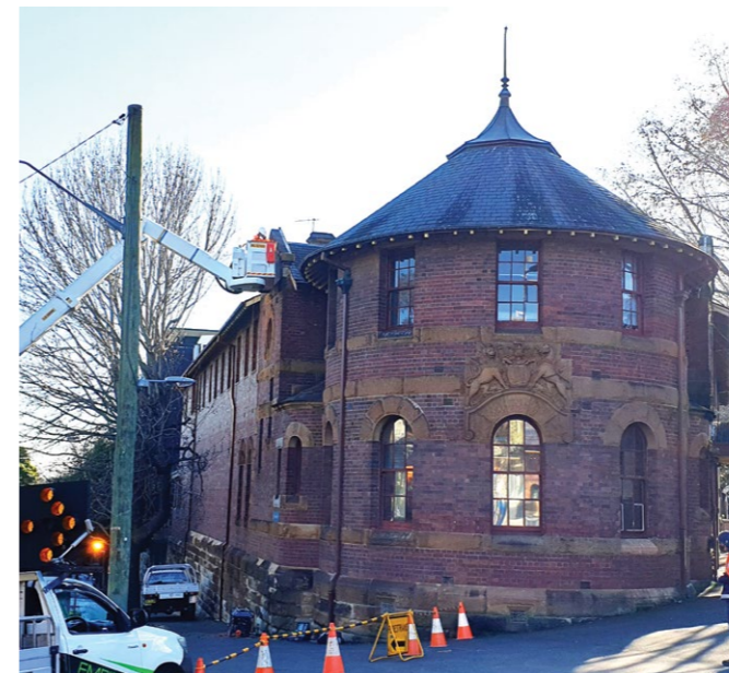
Top left image: Building B Leichhardt Public School condition audit. 35kgs of loose stone was removed during the inspection.
