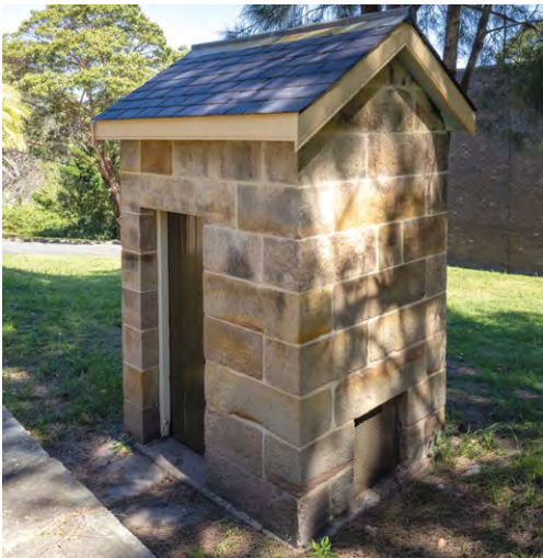
Top: Completed external works Below: Outbuilding
