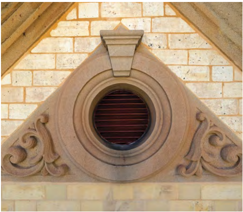
Top: Work underway to repair slate roof Below: Vent and decorative surround Right: Replacement carved detailing
