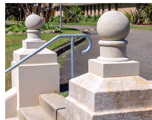
Top: Formal entrance following work
