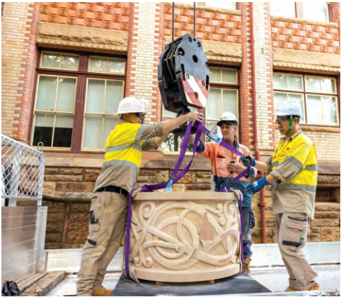
Top: Replacement carvings being installed
