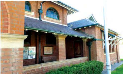
Top image: Construction underway Lower image: Moree Courthouse prior to works
