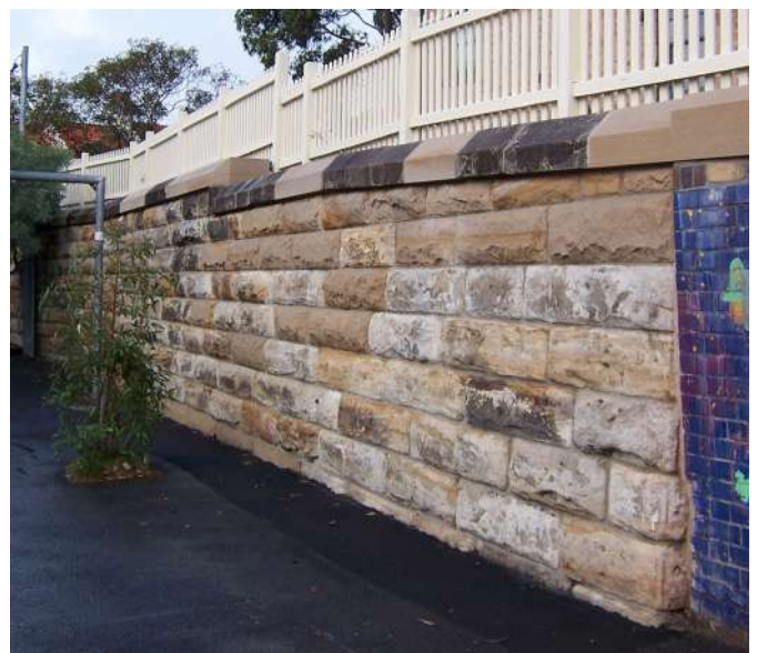
Repaired sandstone retaining wall at completion of works.
