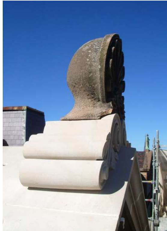
Original acroteria pinned into new apex stone.
