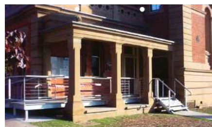
Insertion of ramp to recently conserved portico at Singleton Court.
