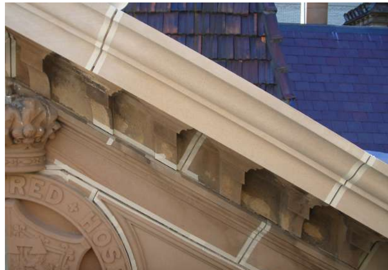
RPA pediment prepared for repointing of joints.
