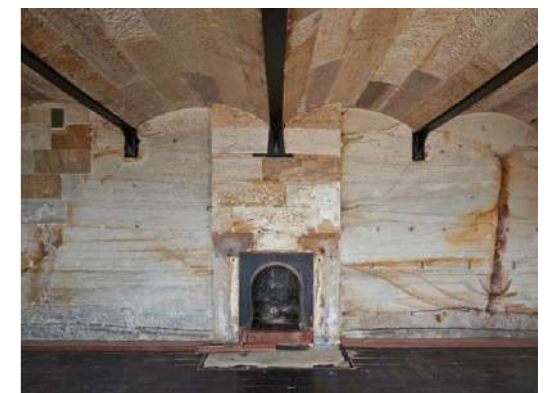
Top image: Stonework revealed: cleaned, desalinated and repointed where required.
