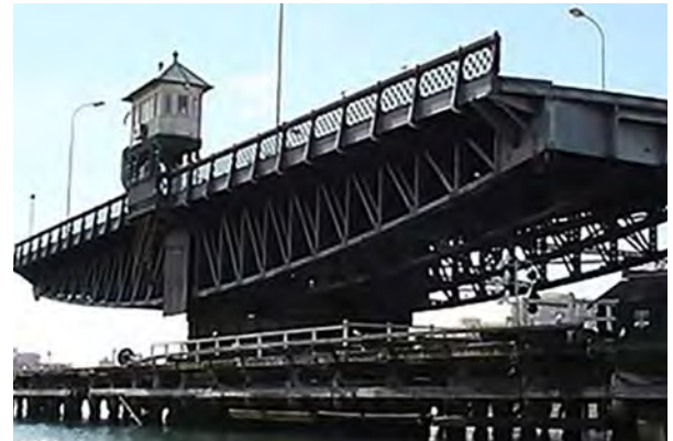
The elevation of the Glebe Island Bridge showing pivot, rest and buttment piers, as well as the delightfully curved central swing span.
