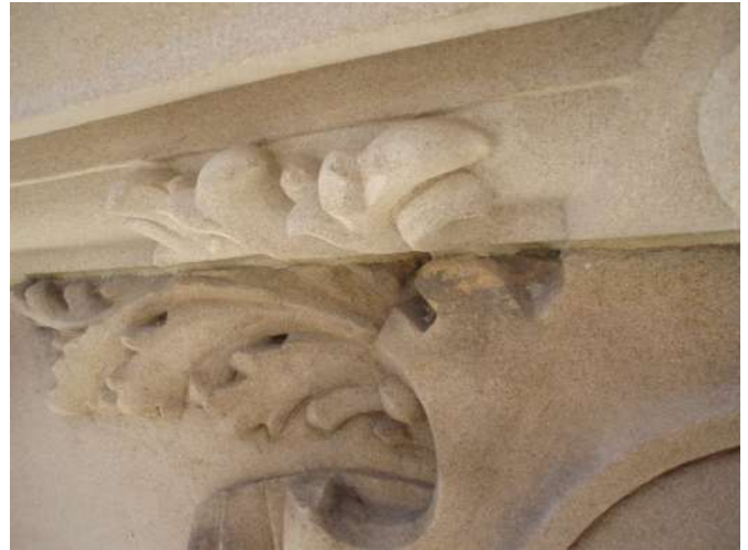
Recarved floral motif adjacent to cartouche over the corner entrance to the Former Ultimo Post Office
