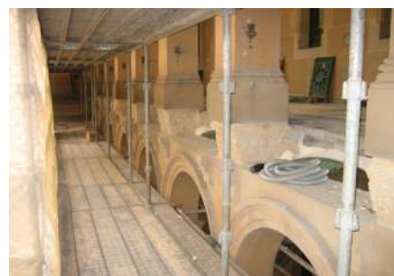
Sydney Hospital Work Area 13, cornice stones removed during construction
