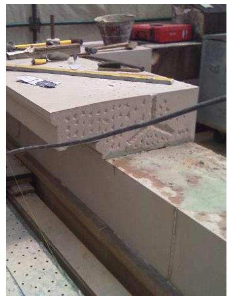
Darlinghurst Courthouse new cornice stone replacement
