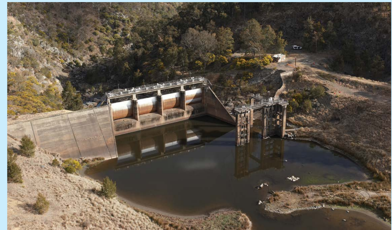
Above: Oaky River Dam, Wollomombi
