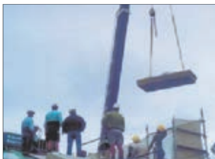
Lifting a new coping stone from College Street.
