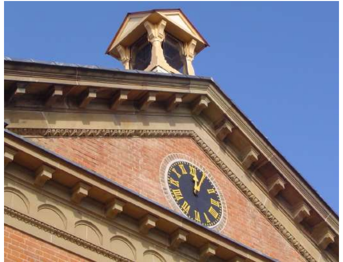
Completed pediment on Elizabeth Street.
