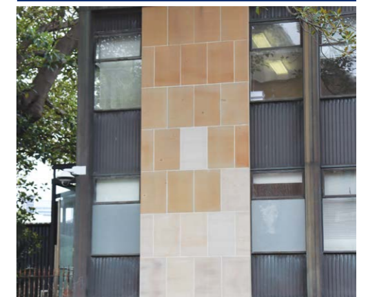
Top image: Completed external conservation works
