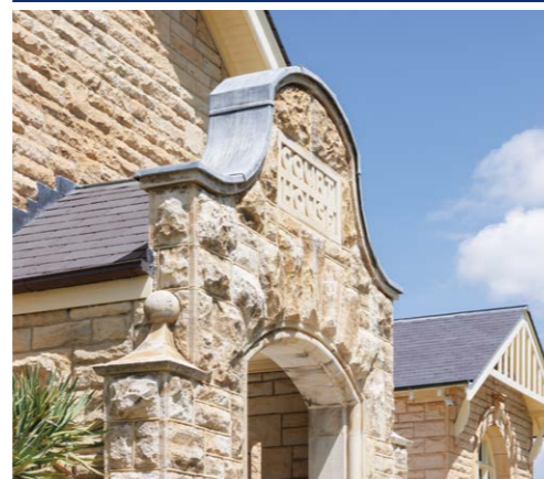
Top image: Completed external conservation works
