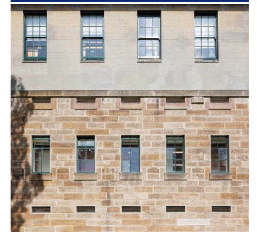
Top image: Completed external conservation works
