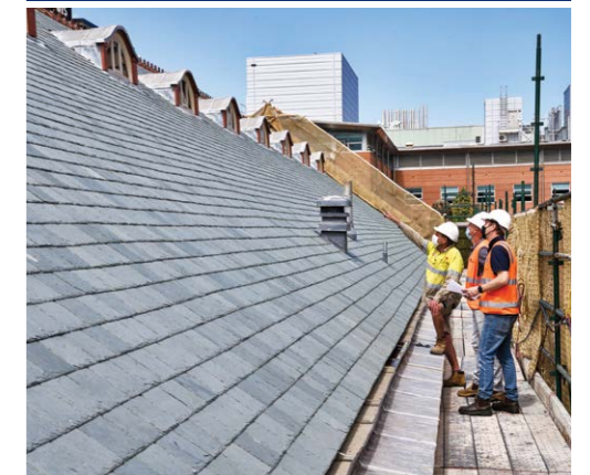
Top image: Completed external conservation works
